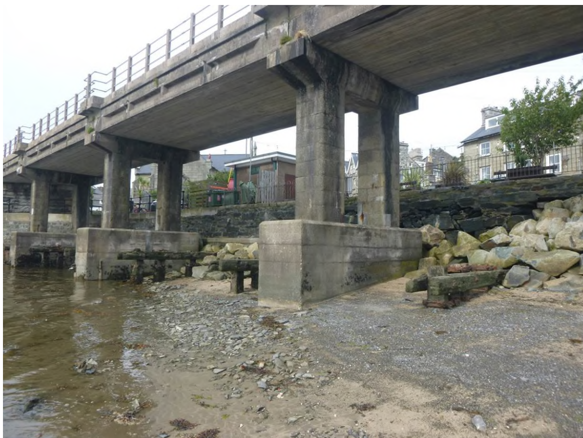
5. Western extent of frontage wall.
