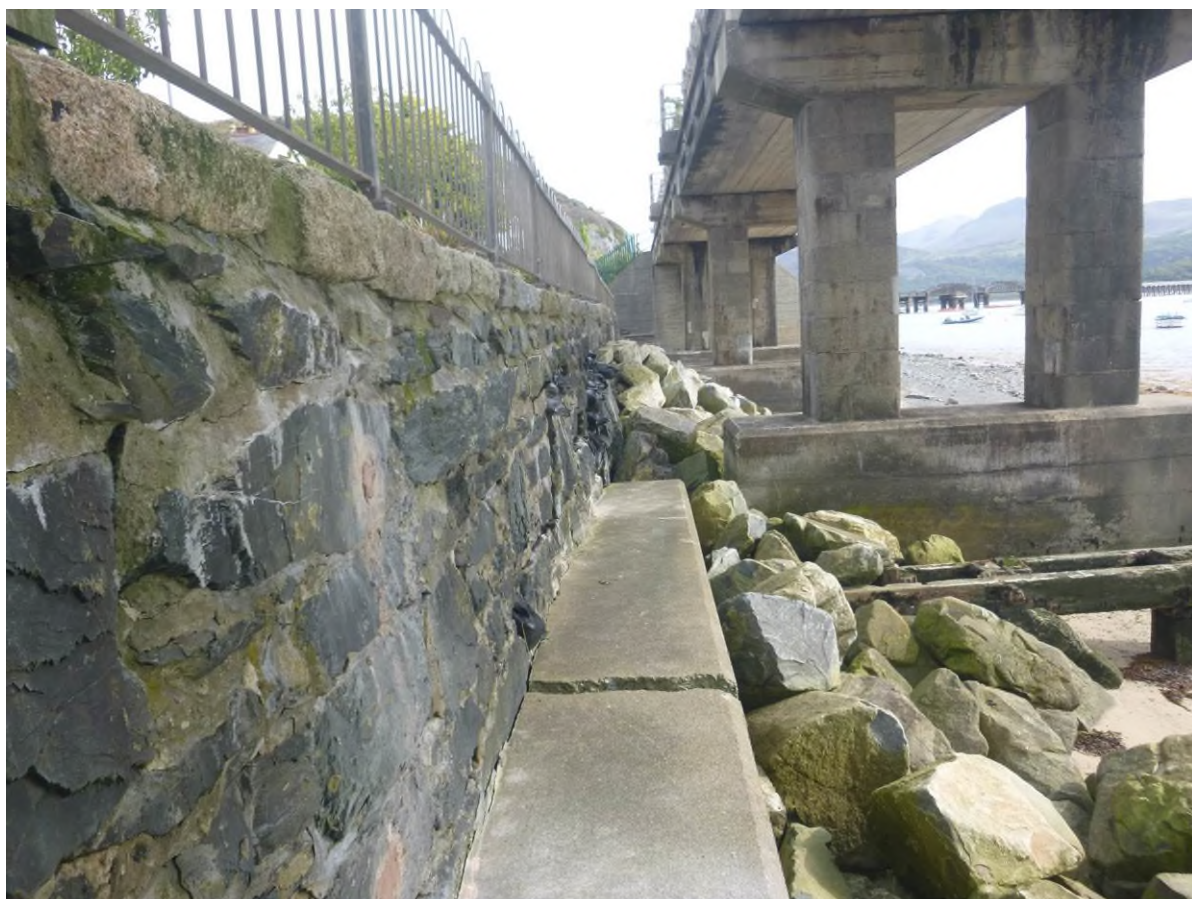
9. Looking east along frontage wall
