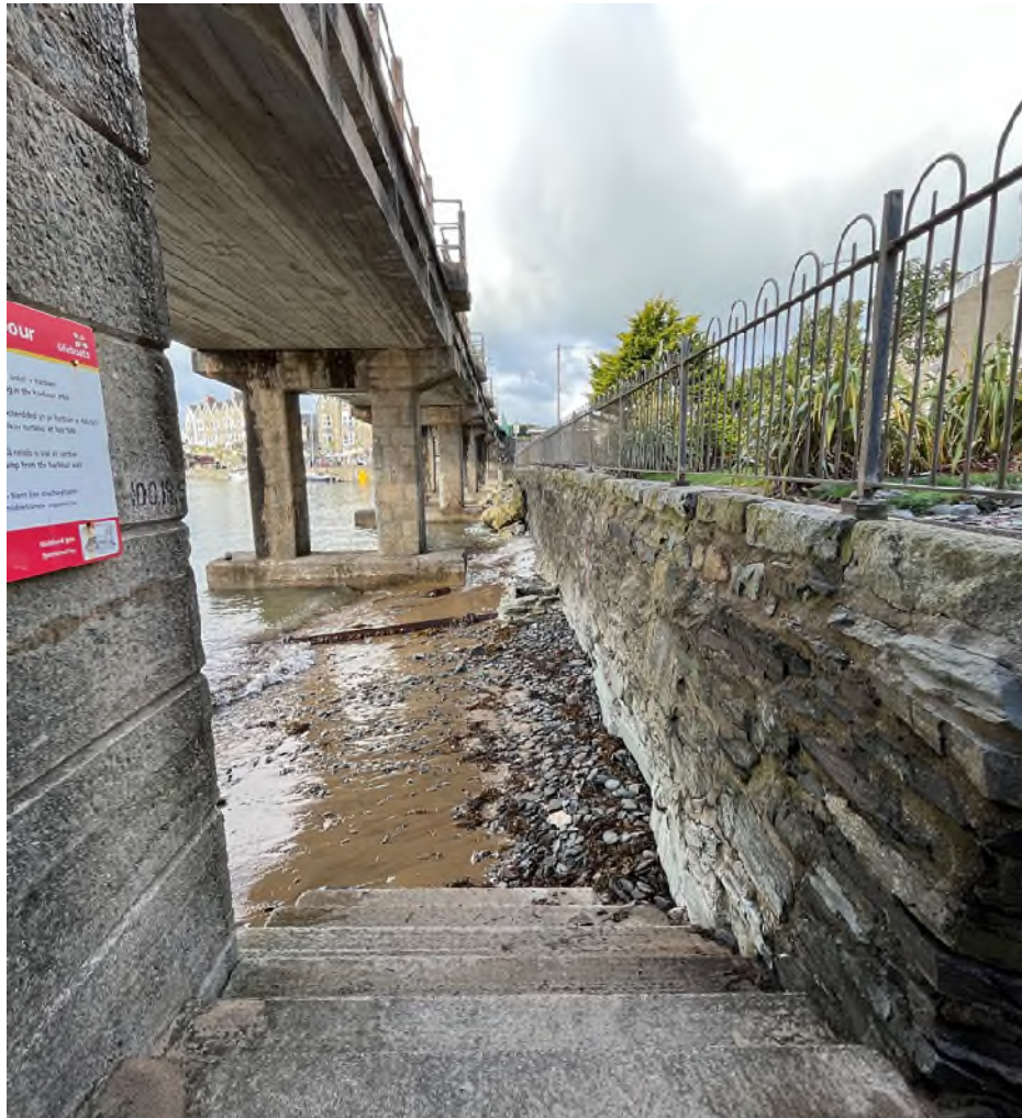
1. Viaduct Gardens frontage wall, looking west across the proposed works area.
