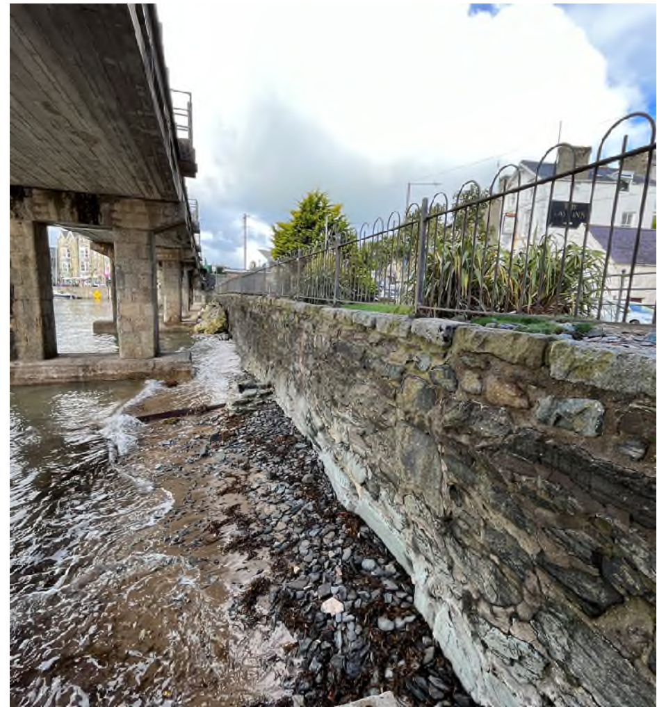
2. Looking west across the proposed works area.
