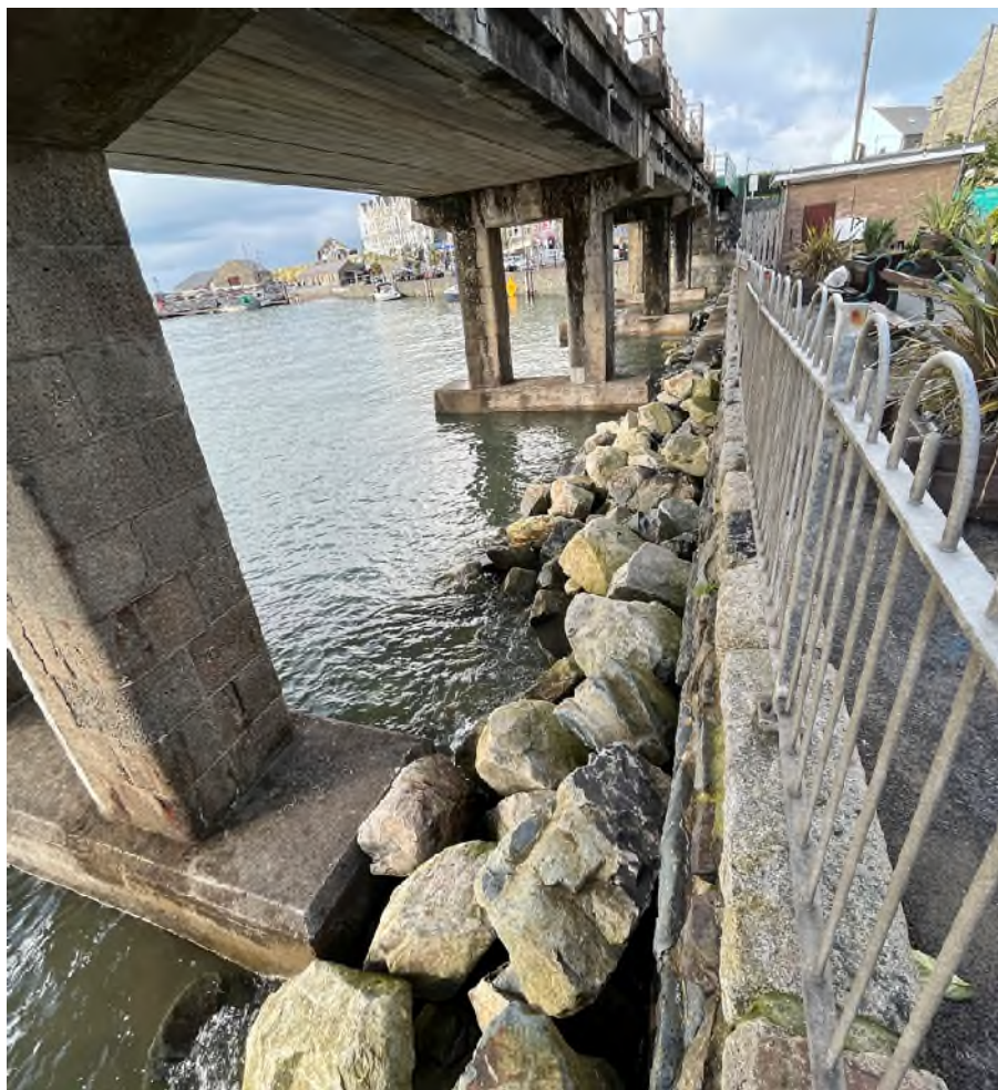
3. Looking towards the western extent of the works area.
