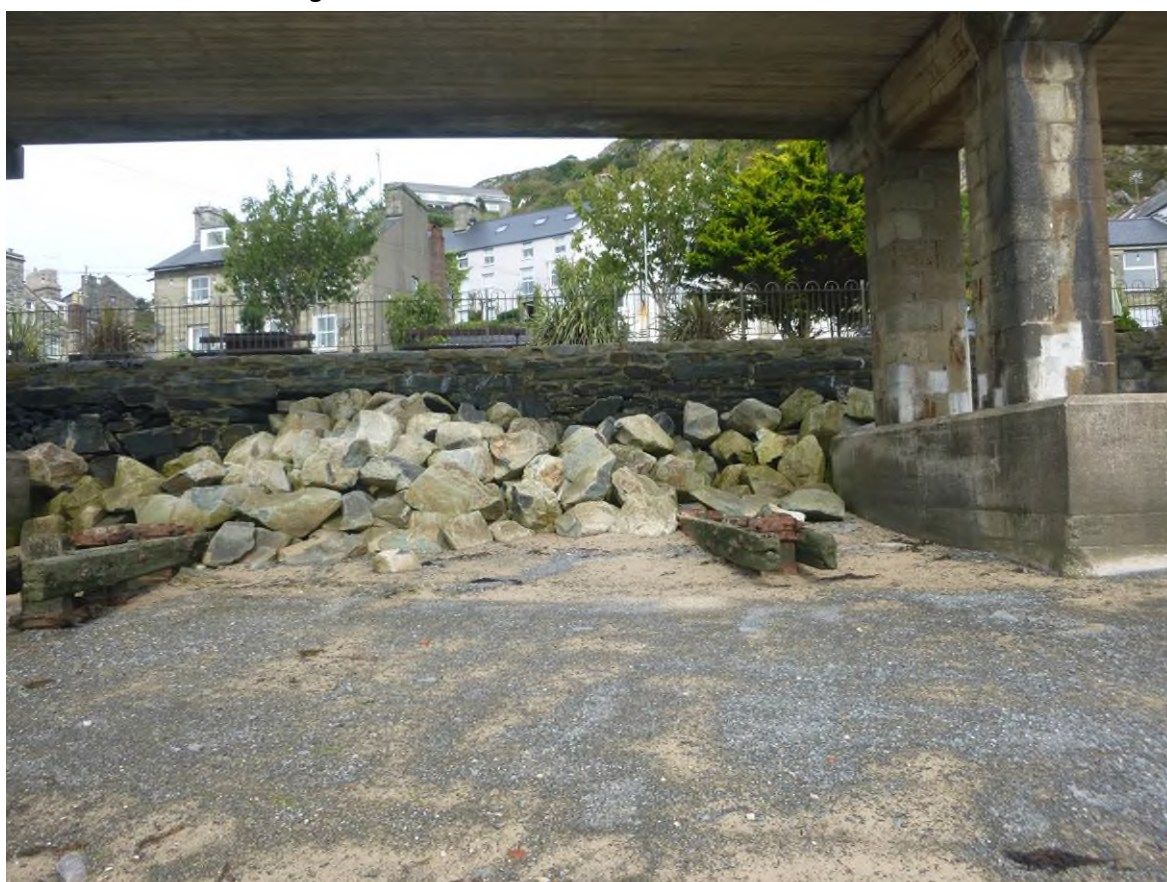
6. Central section of frontage wall
