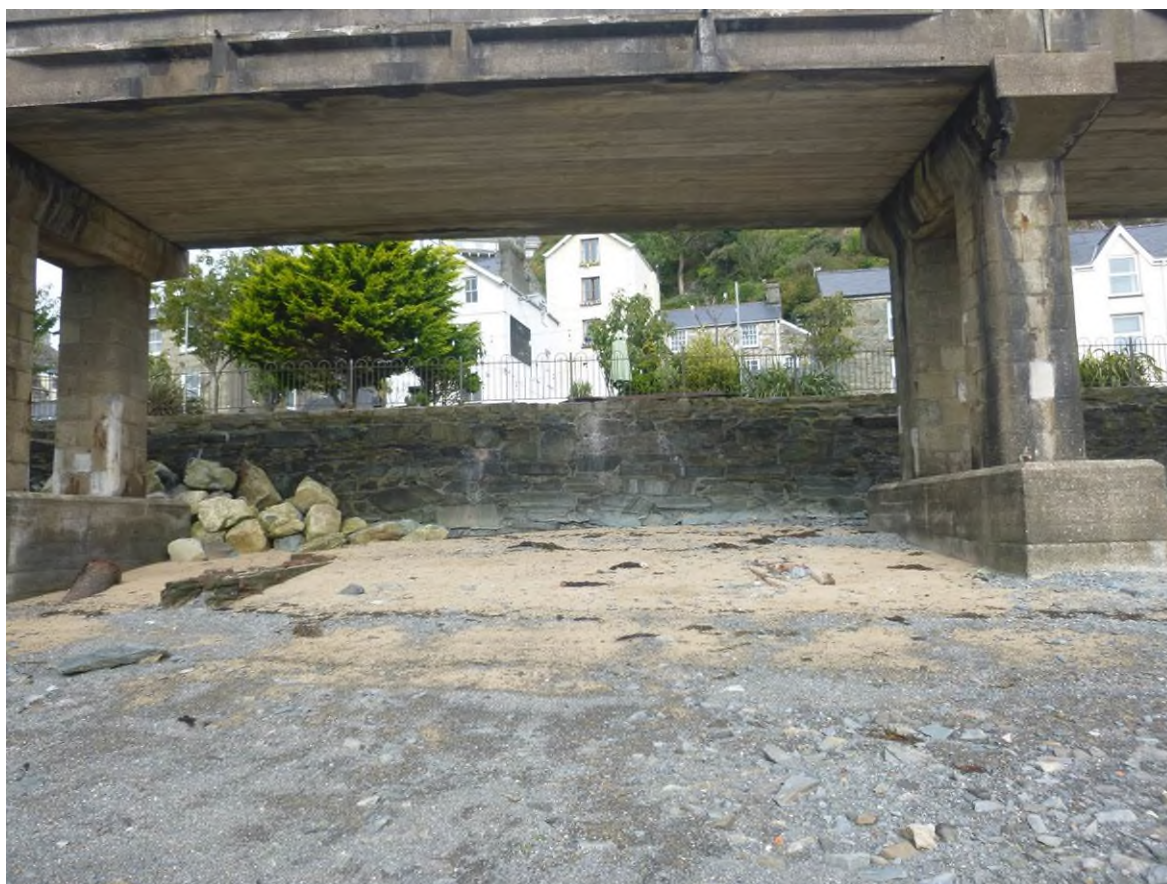
7. Central section of frontage wall
